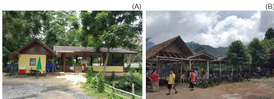
Fig. 3 Permanent buildings Thai Massage Building (A); Permanent buildings Resting pavilion in front of the Community Energy Learning Center building (B)
